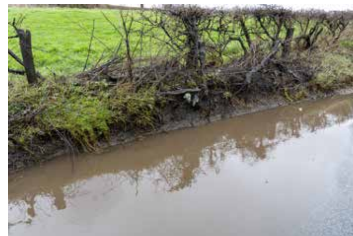
Excess rainfall this Winter has caused roads to flood
